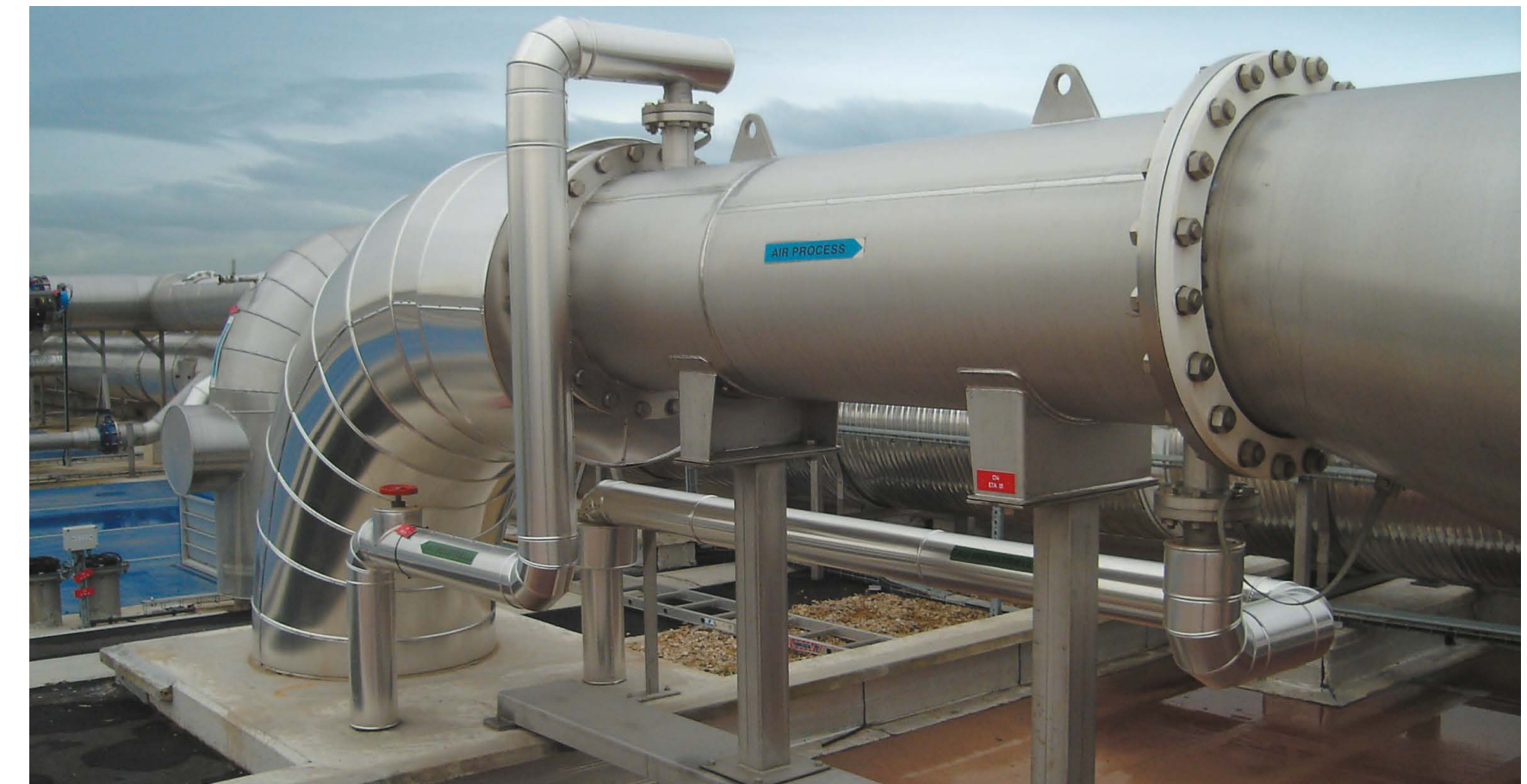
Stainless steel sewer pipe system Picture courtesy of Ugitech GmbH, Renningen, Germany
